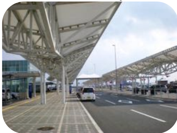
Kitakyushu Airport Membrane roof over walkway
