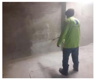
THE CHALLENGE FOR THIS PROJECT WAS TO PREVENT GROUNDWATER PENETRATION THROUGH THE EXISTING BELOW-GRADE WALLS. WATER WAS ENTERING THE INTERIOR OF THE BUILDING DUE TO FAULTY/DEFECTIVE WATERPROOFING THAT HAD BEEN INSTALLED ON THE EXTERIOR OF THE WALL WHEN IT WAS CONSTRUCTED.
