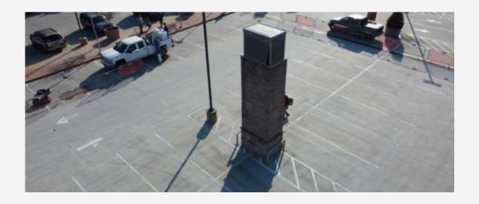
COMMERCIAL RETAIL PARKING LOT WITH BELOW GROUND PARKING WAS EXPERIENCING SIGNIFICANT LEAKING DUE TO CLIMATE AND LOAD BEARING. FIVE PHASES WERE COMPLETE WITH TECHCRETE WATERPROOFING SYSTEM INCLUDING CRACK AND VOID APPLICATION. A RILEM TEST WAS PERFORMED IN TWO TREATED AREAS WHERE IT SHOWED NO ABSORPTION OF WATER.
