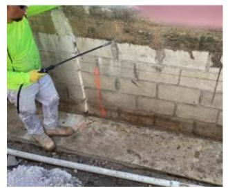
NEW CONSTRUCTION RETAINING WALL INSTALLATION APPLICATION. COMPLETED SEPTEMEBER 2023, TECHCRETE 2500 SYSTEM USED INCLUDING DURATITE FOUNDATION, DURATITE MLASTIC, AND ACR POLYSEAL SEALANT S+.
