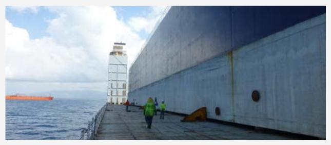
THE LARGEST FLOATING DRY DOCK IN AMERICA NEEDED PROTECTION AND WATERPROOFING DUE TO DIRECT CONTACT WITH SALT WATER AND WEATHER, PREVENTING DETERIORATION OF THE CONCRETE. TECHCRETE 2500 WAS SPECIFIED ON THIS STRUCTURE.
