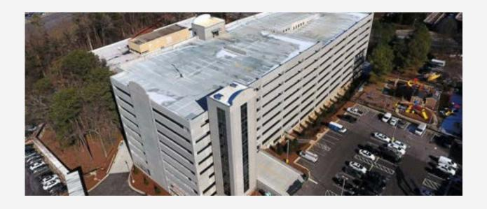
HOSPITAL PARKING RAMP WATERPROOFED IN 1999. THE ENGINEER ON THE PROJECT (SEDKI & RUSS) OPTED TO USE OUR SPRAY-ON FORMULA INSTEAD OF THEIR NORMAL POLYURETHANE 'TRAFFICABLE MEMBRANE' BECAUSE THEY BELIEVE 'MEMBRANE' AND 'TRAFFIC' ARE NOT COMPATIBLE.
