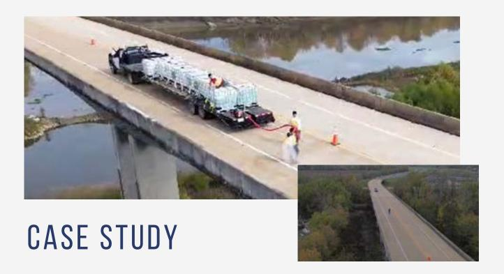
BRIDGEDECK WATERPROOFING SYSTEM WAS SPECIFIED TO PROTECT THIS BRIDGE ON INTERSTATE 20. THE INTERSTATE WHICH WAS CONSTRUCTED IN 1957 NEEDED PROTECTION AGAINST ENVIRONMENTAL AND CHEMICAL ELEMENTS TO PREVENT INGRESS OF CLORIDE IONS AND CORROSION.
