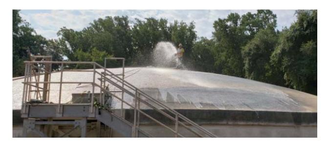
WATER STORAGE TANKS BUILT IN 1957, WITH DOMED ROOFS MADE OF STRUCTURAL CONCRETE WHICH STORE A COMBINED TOTAL OF 6 MILLION GALLONS OF POTABLE WATER. OVER THE YEARS, THE CONCRETE TANKS HAD DETERIORATED TO THE POINT WHERE SEVERAL HUNDREDS OF THOUSANDS OF DOLLARS OF REPAIRS WERE REQUIRED. ONCE THE REHABILITATION WORK WAS COMPLETED, TECHCRETE SYSTEM WAS THE IDEAL WATERPROOFING SOLUTION.
