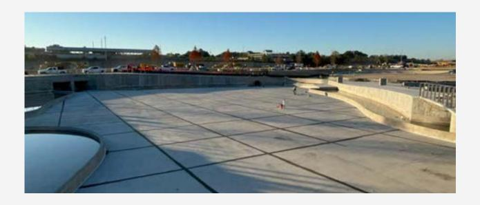
NEWLY CONSTRUCTED FILMING STUDIO WITH 45,000SQFT OF STORM WATER HOLDING & FOUNTAIN AREAS WERE PROTECTED WITH TECHCRETE 2500 WATERPROOFING SYSTEM. THIS SYSTEM ALSO FEATURED A KEY ACCESSORY: DURATITE MLASTIC.
