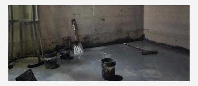
TECHCRETE 2500, A HIGH-PERFORMANCE WATERPROOFING PRODUCT, WAS RECENTLY USED TO SEAL A CONCRETE WATER TANK ON SOUTH BELL STREET. KNOWN FOR ITS ABILITY TO DEEPLY PENETRATE CONCRETE AND CREATE A DURABLE WATER BARRIER, TECHCRETE 2500 WAS APPLIED AFTER THOROUGH SURFACE PREPARATION. THIS APPLICATION ENSURES THE TANK'S LONG-TERM WATER TIGHTNESS AND STRUCTURAL INTEGRITY, ESSENTIAL FOR RELIABLE WATER STORAGE AND DISTRIBUTION INFRASTRUCTURE.
